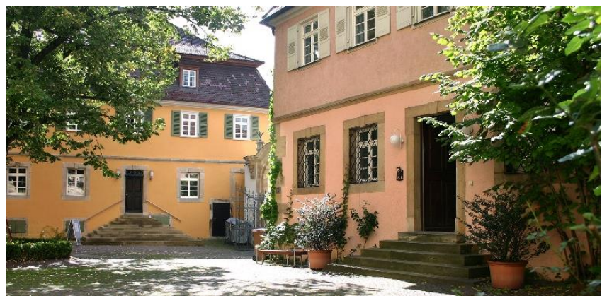
Abb. 1: Innenhof Campus Innenstadt C11
